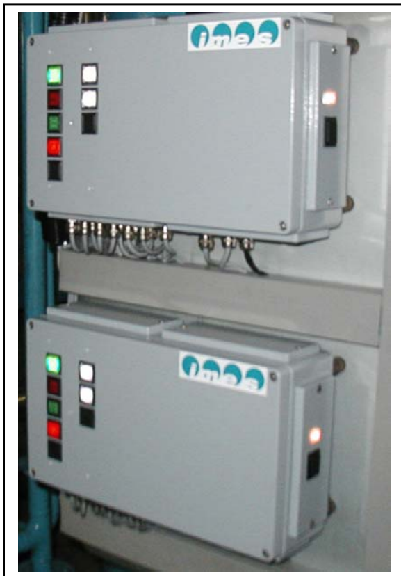
Abb.13: ZAD unit on a 20 cylinder gas engine
